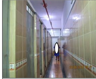
Photo of the sanitary facilities Workers toilet.JPG
